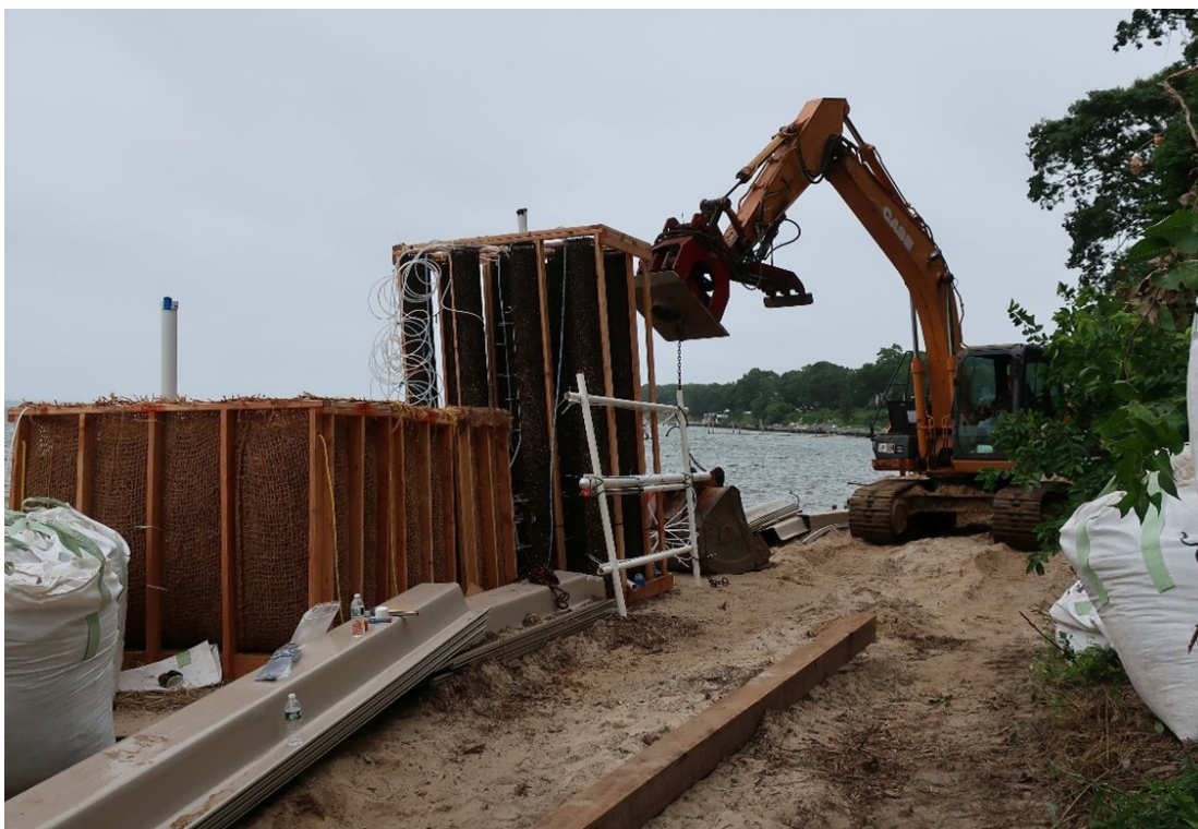
Figure 9. Example of a trench-type and woodchip column array PRB installation using pre-filled frames placed in the subsurface using a traditional backhoe. Photo credit: CCWT.
