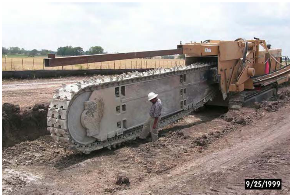
Figure 6. Picture of a deep trencher, which may be needed for PRBs installed between 20 feet and 40 feet below land surface.
