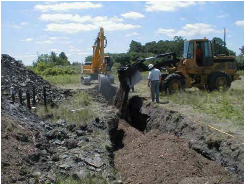
Figure 5. Woodchip PRB installation using conventional trenching equipment.
