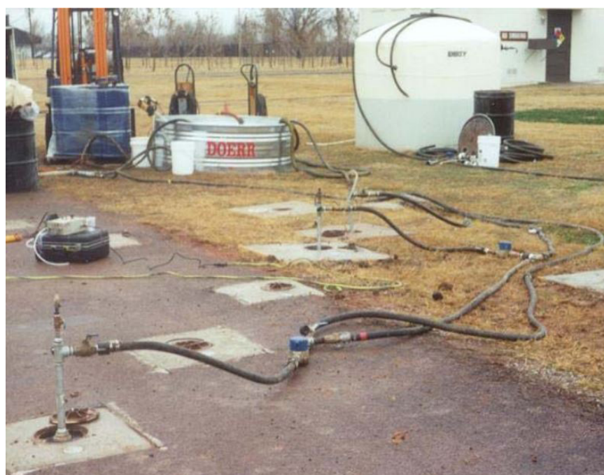
Figure 7. Emulsified Vegetable Oil Injection at Environmental Remediation Site.
