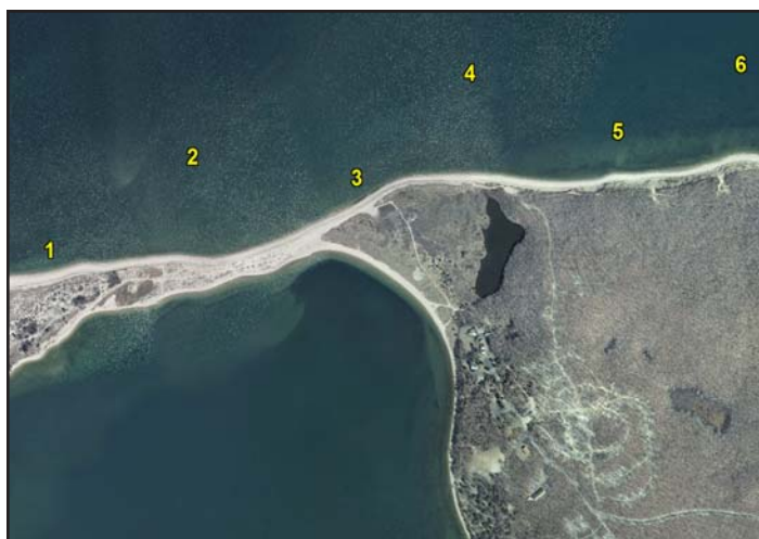
Figure CP-1. An aerial view of the Cedar Point monitoring site with monitoring stations indicated by the superimposed numbers.
