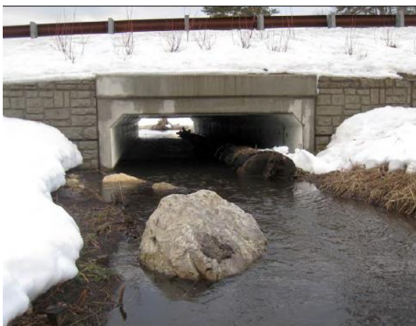
Figure 23: An example of a concrete box culvert with natural channel substrate on the bottom and a floodplain bench built for terrestrial organism passage.
