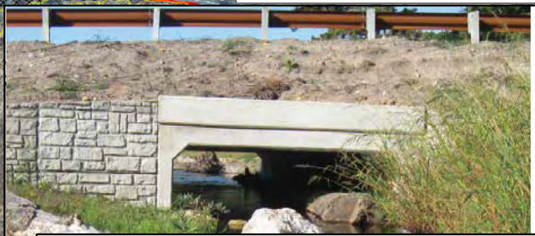
Example photo and sketch of a box culvert with natural bed substrate (courtesy of Resilient Crossings Handbook)
