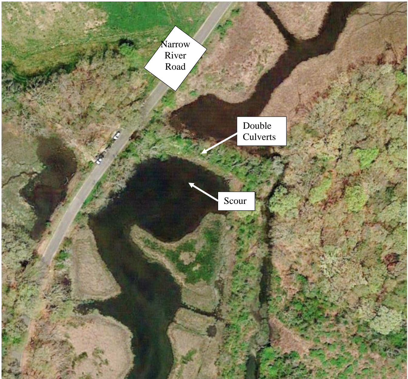
Figure 17: Scour and erosion upstream and downstream of the double culvert.
