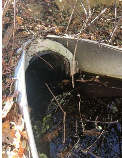
Figure 4: Culvert at Route 25 crossing.
