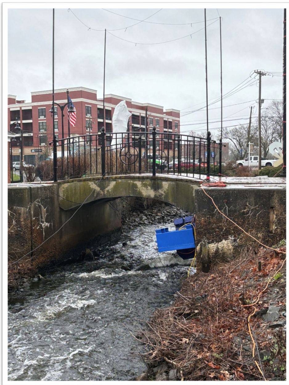
Figure 1. Camera box vandalized at Grangebél, all equipment was pushed over the walkway during heavy rain and some parts were submerged.
