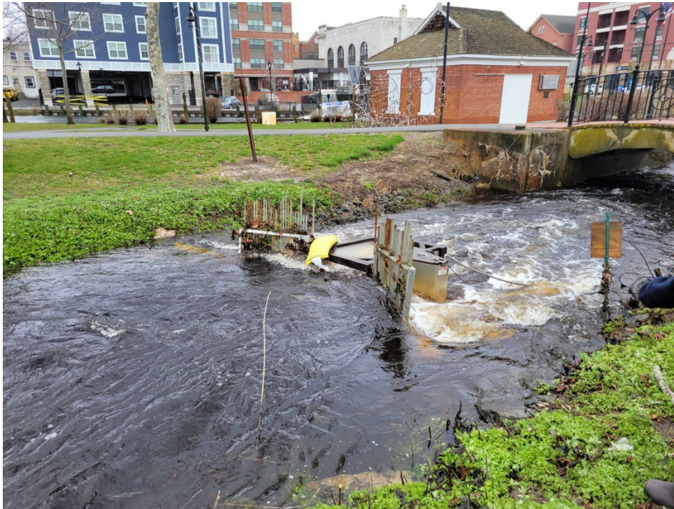
Figure 1. Image of Camera box during high water level, showing passage ability around weirs. Note the eroding banks on either side of the weir.
