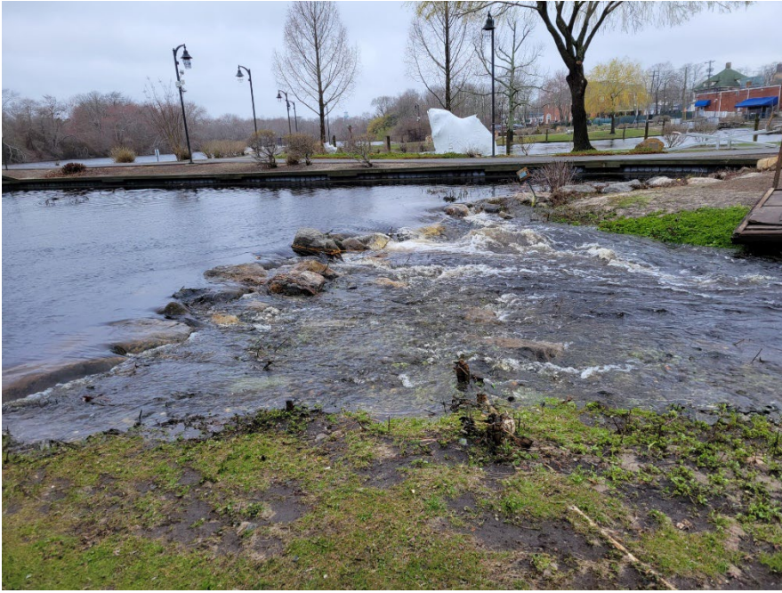
Figure 2. Upstream Exit in Grangebel Fishway during flooding event; RFID antenna completely submerged.
