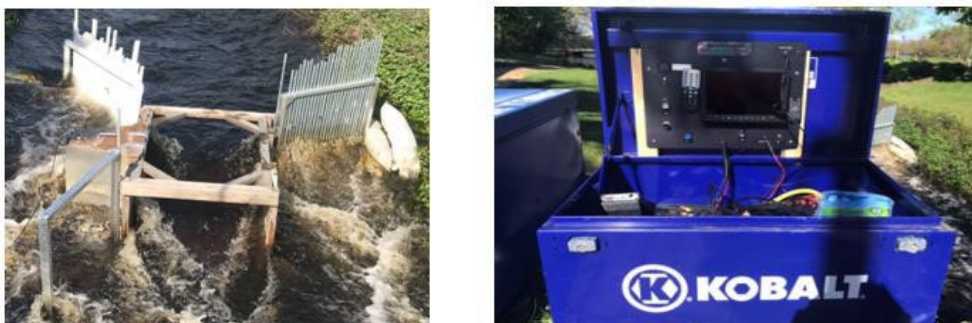
Figure 4 – Video monitoring set-up at the Grangebel Park fishway (left) and site job box (right)
