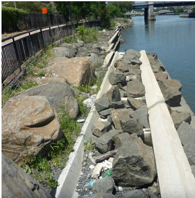
Looking north: Hard structural features along the shoreline composed of cement baskets filled with rip rap.
