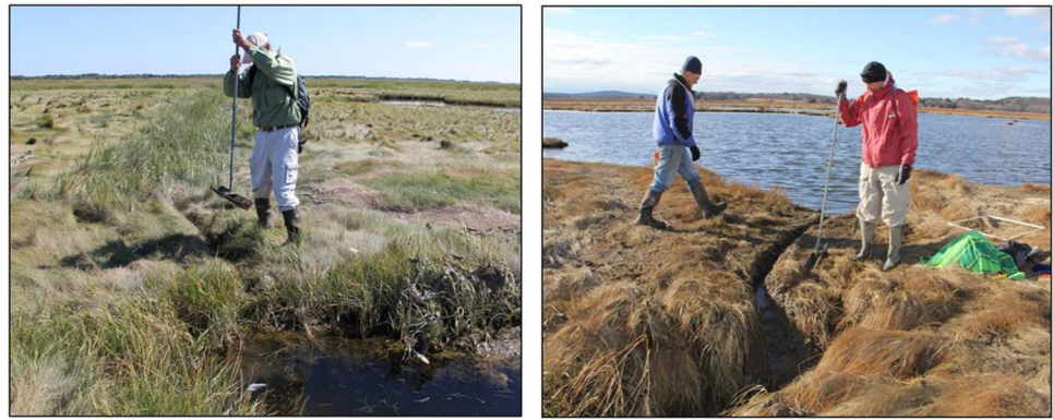
Fig. 2 Left: Creation of runnel by compacting the marsh surface using a handheld tamping tool at the north pool site in 2015. Runnel connected an existing ditch to the expanding pool. Right: Runnel at the south pool site in 2015 after construction. Runnels were created with dimensions of approximately 30 cm width - 15 cm depth and lengths of 60 – 200 cm
