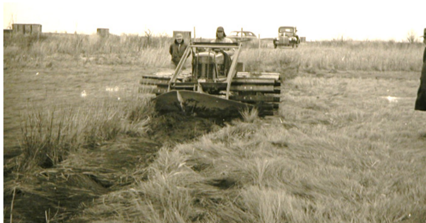
FIGURE 9. Scavel plow clearing debris from a mosquito control ditch circa 1940-1950s. Mechanized ditching patterns are ubiquitous from Massachusetts southward, often overlay previous agricultural ditching patterns, may not adhere to tideshed boundaries or original marsh slope, and develop highly compacted embankments on both sides of ditches. (Photo credit CT DEEP.)
