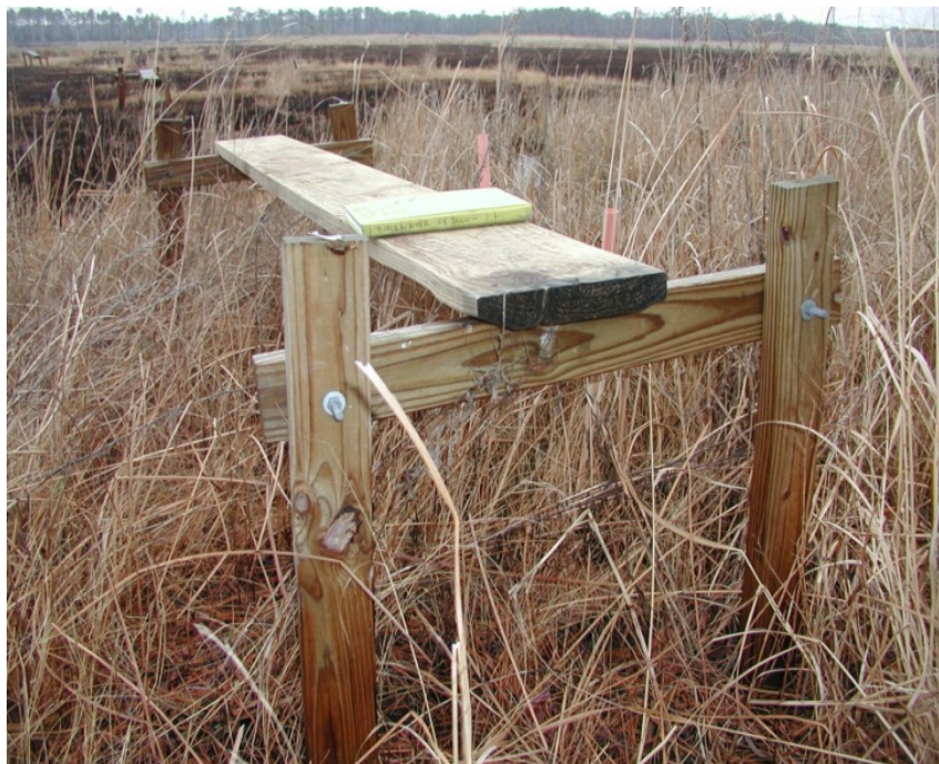
Figure 2.11. Installed platform (Blackwater NWR, MD USA).
