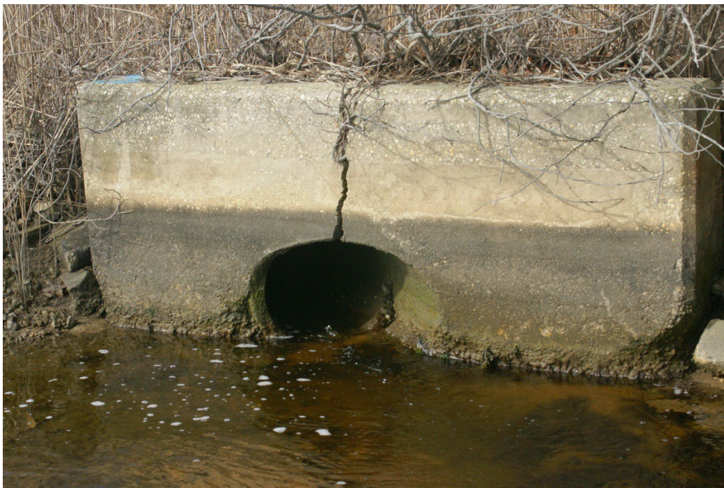
Photo 5 - Headwall on South Side of Route 25 Culvert
