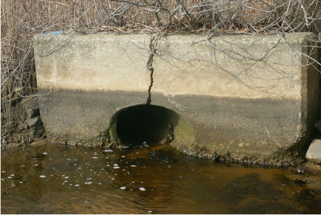
Photo 5 - Headwall on South Side of Route 25 Culvert
