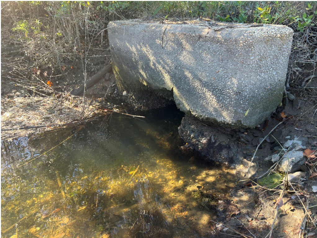
Photo 8 - Headwall on South Side of Old Main Road Culvert
