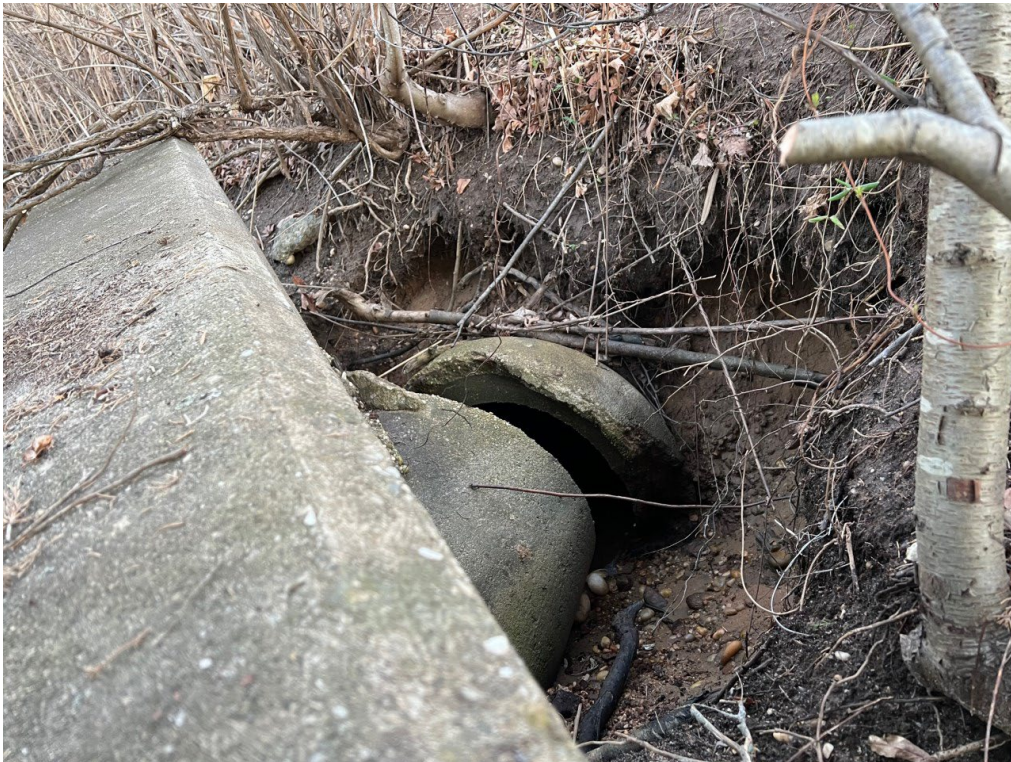
Photo 4 - Failed Headwall on North Side of Route 25 Culvert
