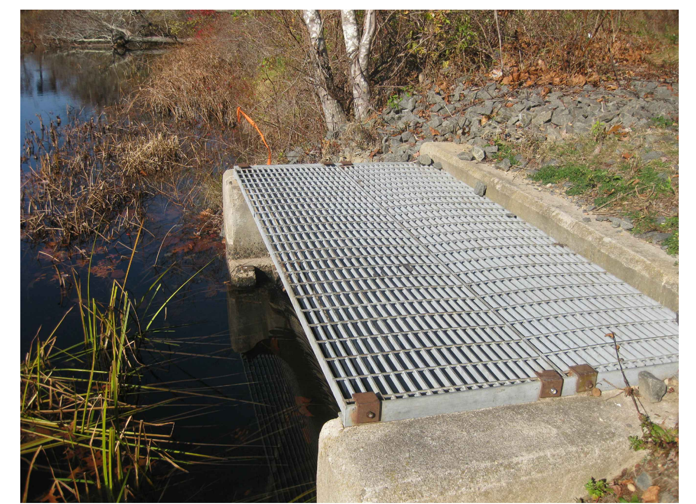
PHOTO 4: EXISTING INLET STRUCTURE
