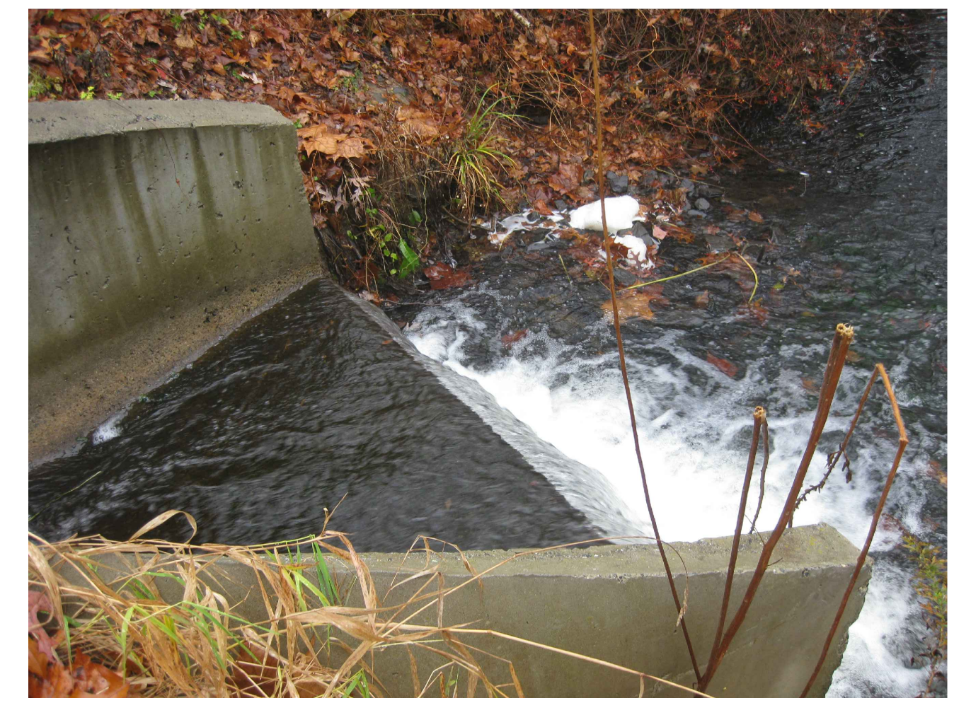
PHOTO 5: EXISTING OUTLET STRUCTURE
