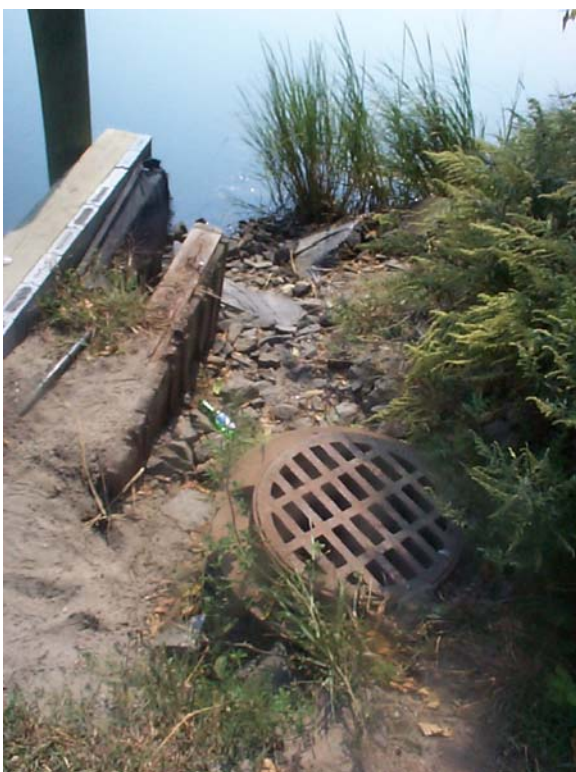
MH-4 Manhole Erosion
