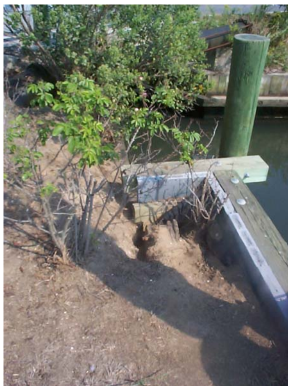
MH-4 Retaining Wall Erosion
