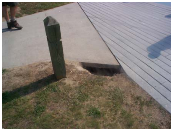
MH-4 Sidewalk Erosion
