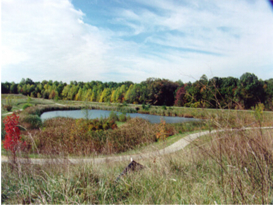
Example of a wet retention pond (Source: Maryland Department of the Environment, 1999)
