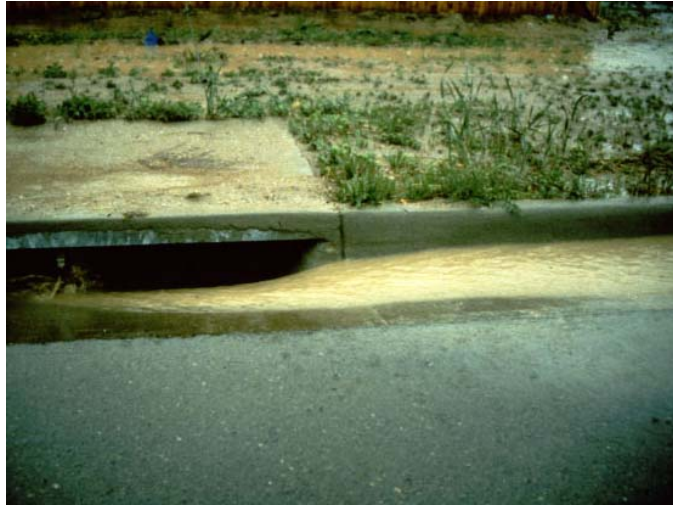
Runoff from a construction site entering a storm drain inlet illustrates the need for inlet protection (Source: Center for Watershed Protection, 2001)
