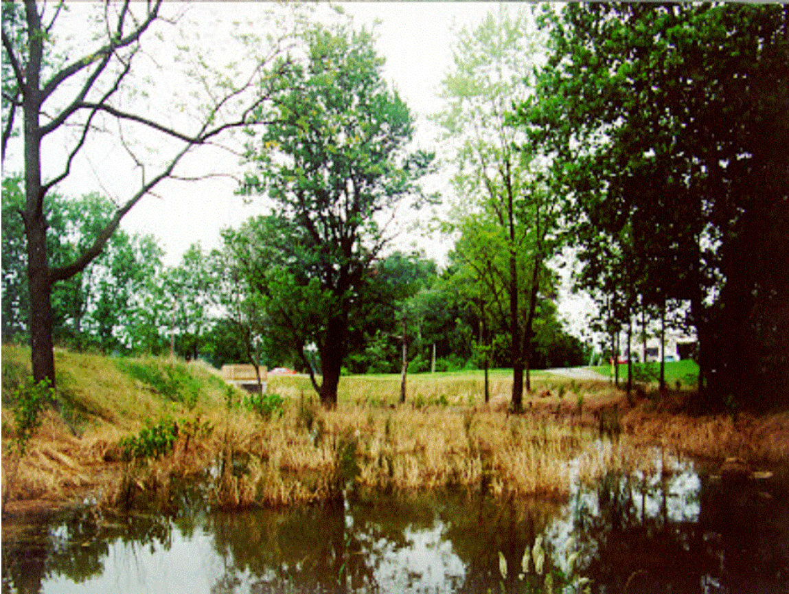
Example of a constructed stormwater wetland (Source: Galli, 1997)
